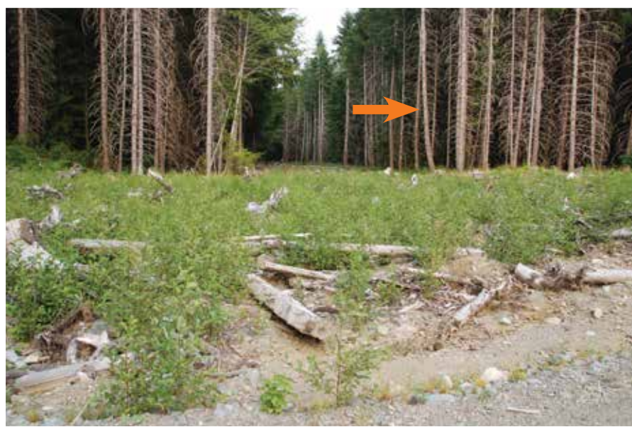
Figure 3. Heber Dam penstock right-of-way following 3 years of vegetation growth.
